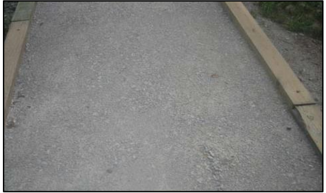
3/4" limestone with 50% dust after two lifts installed and compacted
