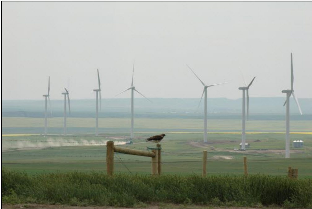
Wind turbine farm west of Magrath
