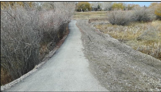
Looking north at recent bank stabilization work adjacent to trail
