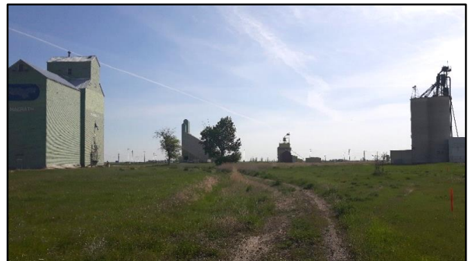
Picture 48 - Looking east from segment 22 at "elevator row" from 3 rd Street W
