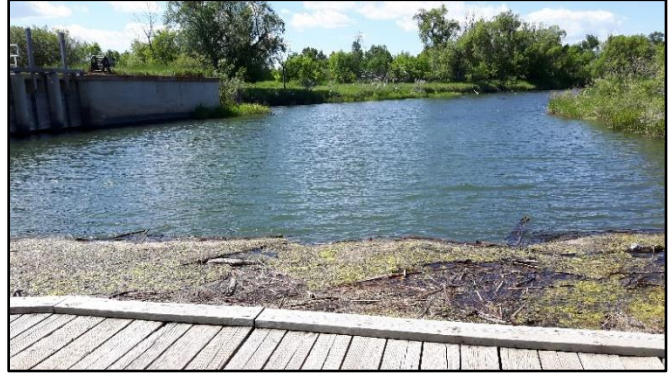
Looking west upstream of Magrath Irrigation Headworks
