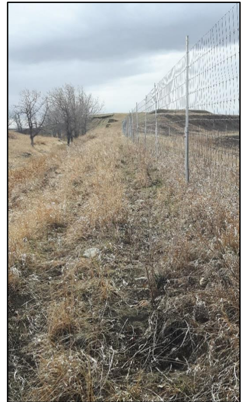
Picture 14 - Looking southwest along former irrigation canal bank within segment 10
