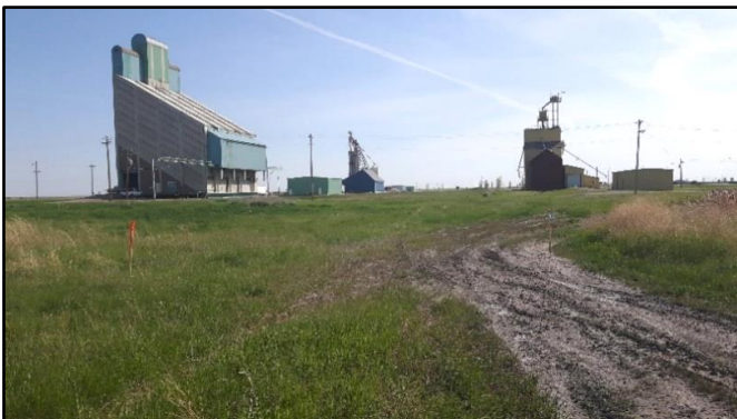
Picture 47 - Looking northeast from segment 22 at "elevator row"
