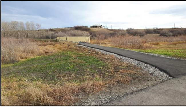
Looking northeast at new bridge (August 2016) over Pothole Creek
