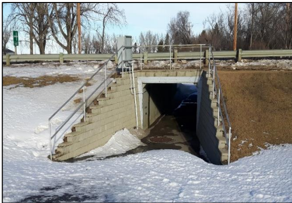
Tunnel for golf cart/walking path beneath Highway 534 (Vulcan, AB)
