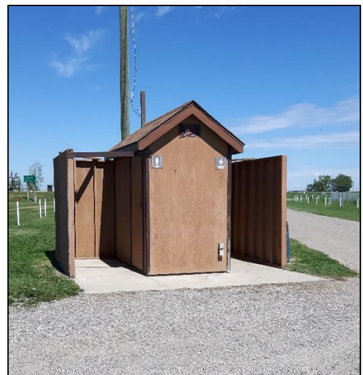
Existing washroom facility in Cook Centennial park
