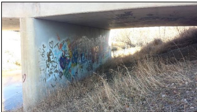
Picture 2 - Looking east below Highway 62 bridge at segment 3
