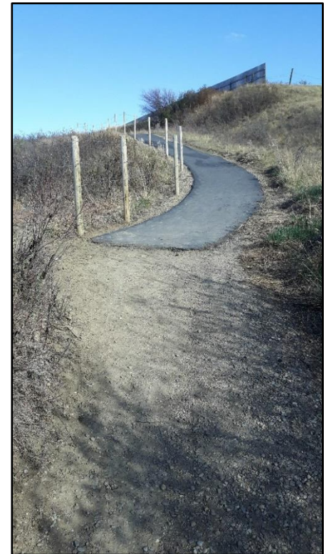
Existing gap in pavement (paved in August 2016) adjacent to Magrath Golf Course
