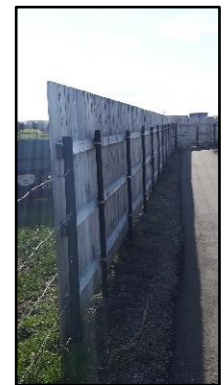
Board fence on outer loop of existing trail
