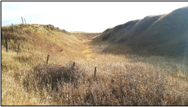
Picture 76 - Looking south at magnificent former irrigation canal located east of Old Raymond Bridge
