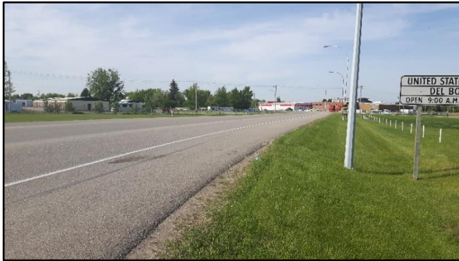
Picture 43 - Looking southwest from potential Highway 62 crossing location within segment 21 adjacent to future wetland area
